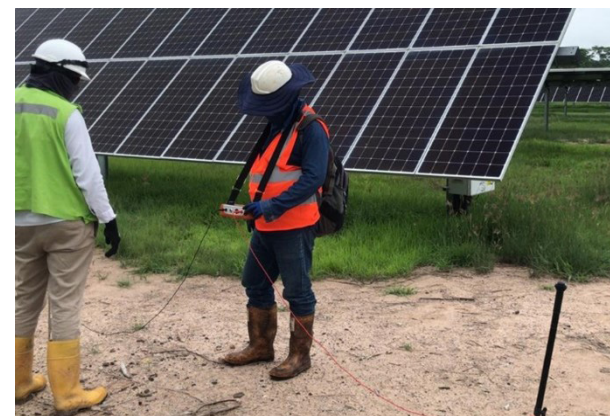
Fig. 2. Pinpointing a fault in buried cable.
