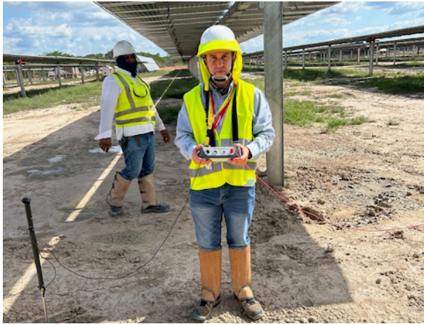
Fig. 4. Pinpointing a fault in buried cable.
