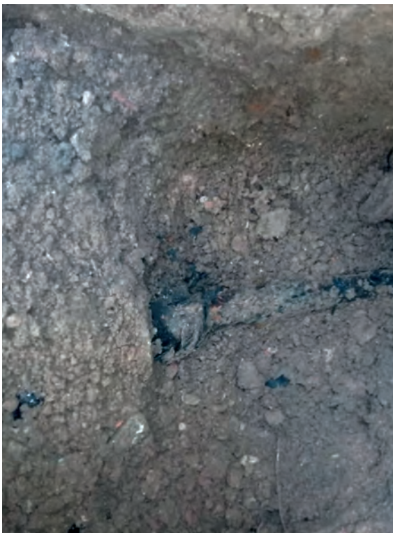
Figure 6: Splice body is located and uncovered
