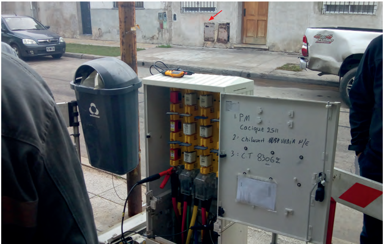
Figure 2: Typical residential three-phase fuse cabinet
