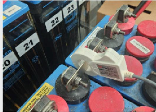
Continue taking measurements of each cell and strap in sequence until you reach the last cell in the string. When the BITE5 ADVANCED measures the last cell in the string, it will display a summary.
