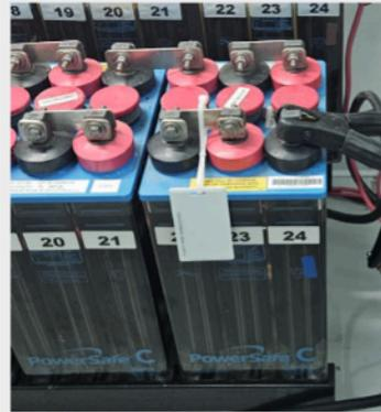
The RFID tag number will now show up on the configuration screen. Now when this tag is scanned this battery string configuration will be called.
